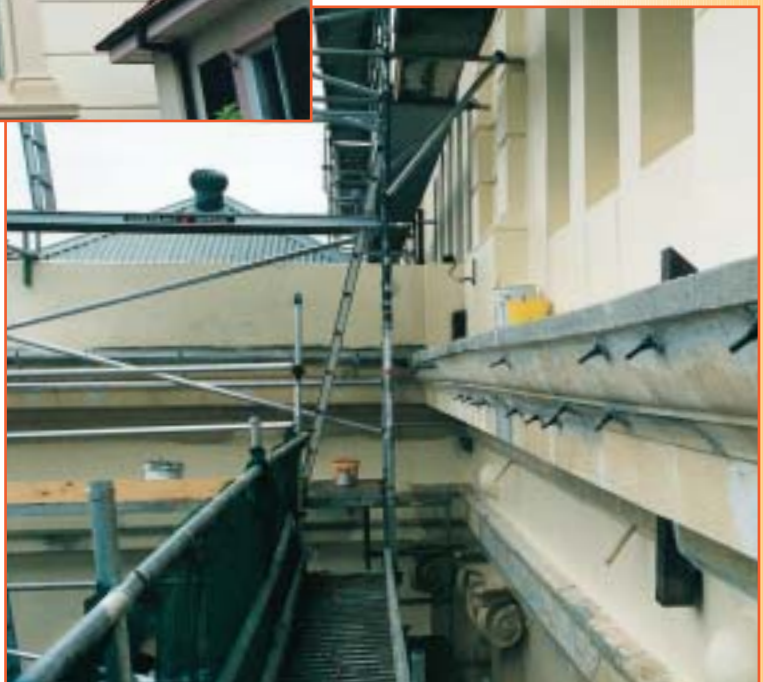
Repair systems being placed using Sika MonoTop-615HB and Sikadur-52.
