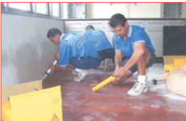
Application of Sikaflex-PRO.
