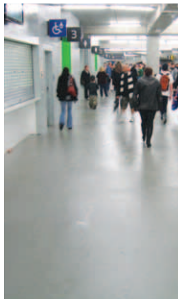
Rectangular Stadium – Melbourne February, 2010 Product – Sikafloor®-2530W and Sikafloor® 2635L/264 Applicator – Abel Flooring
