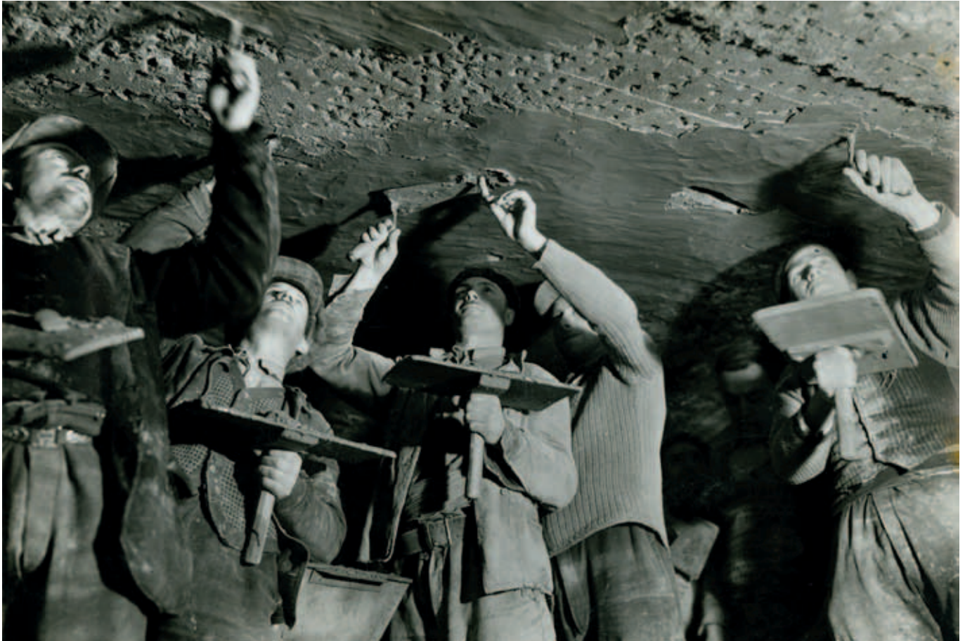
Waterproofing a tunnel in Stuttgart, Germany, 1930
