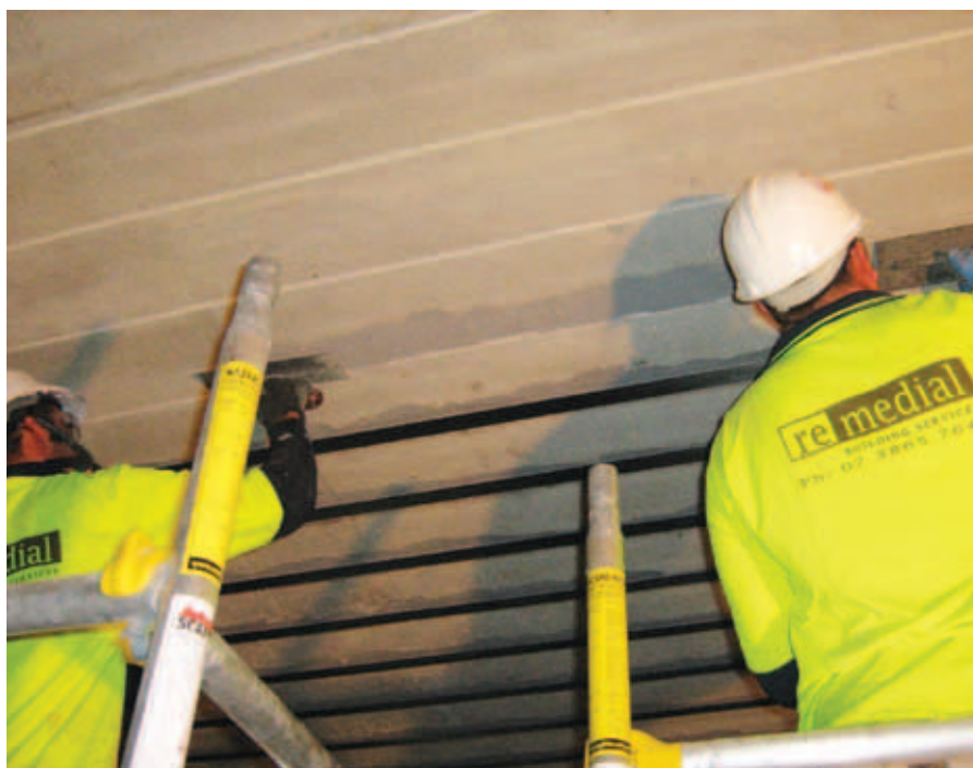
111 Eagle Street, Brisbane Product – Sika CarboDur® and Sikadur® 30 Applicator – Remedial Building Services
