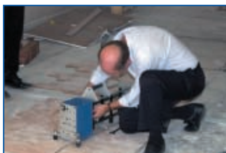
Testing the Sika AcouBond® System
