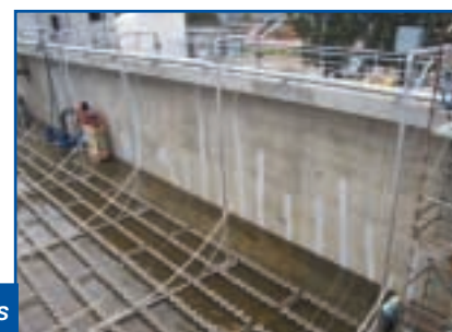
Applying Sikaflex®-Tank
