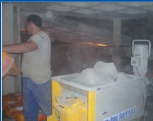
Mixing Sikafloor®-Level 25
