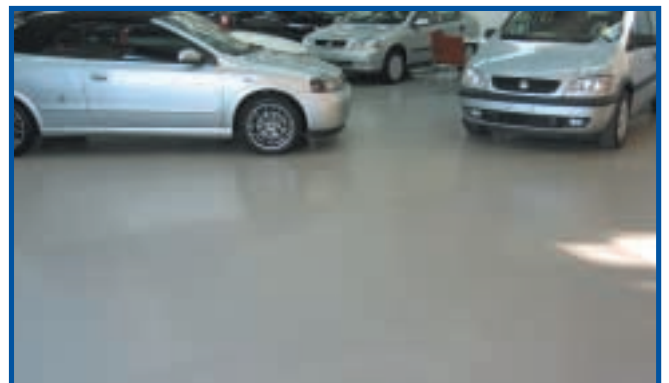
— The finished Sikafloor®-261T floor
