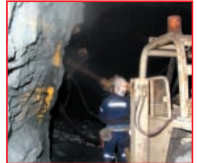
— Spraying in-cycle Shotcrete
