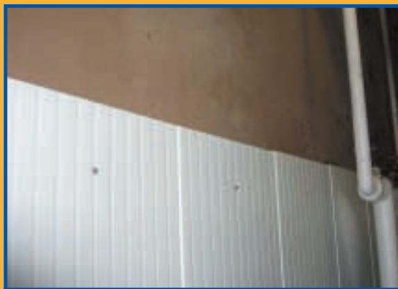
SikaTite-BE covered by cool room panels
