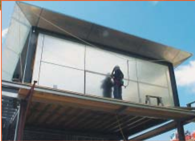
Panel bonding using Sikaflex-252.
