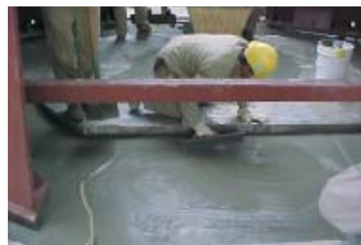
SikaGrout at power plant, Millmerran, QLD.
