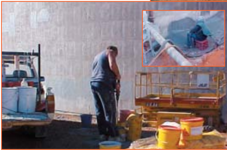
Application of Sika repair materials (inset: Sika Gunite GP).
