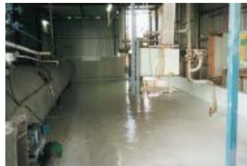
Sikagard in bund, Newcastle, NSW.
