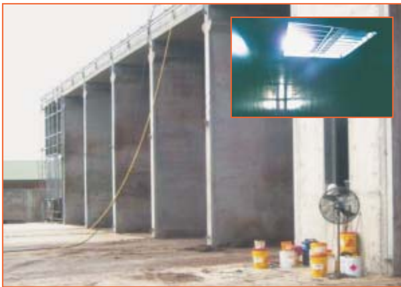
New tanks waiting to be waterproofed (Inset – Sika Tite-BE coated inside).
