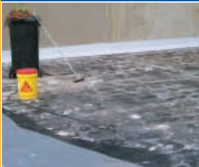
The existing bituminous membrane
