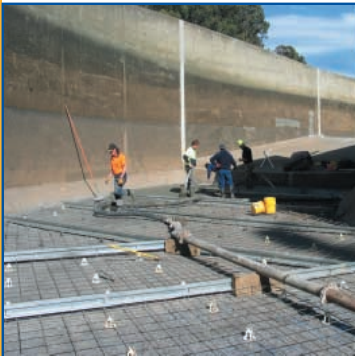
Spillway with previous Sika repairs on walls
