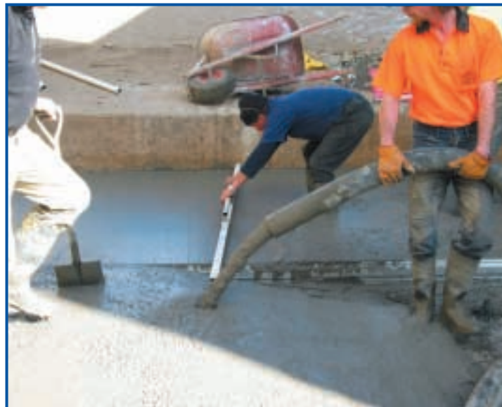
Pumping and screeding of the concrete
