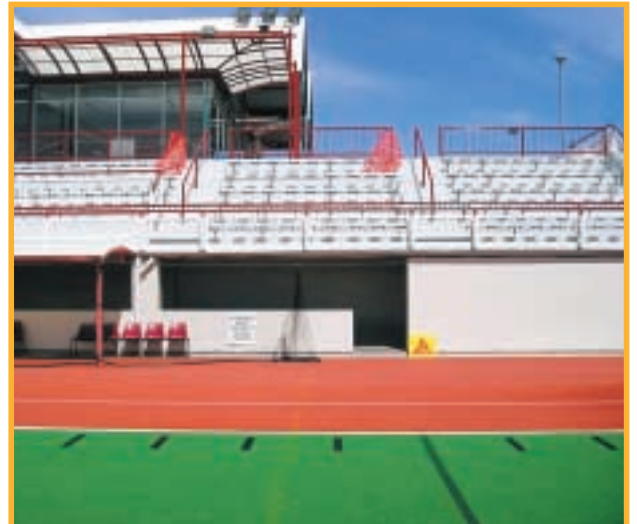
The freshly coated Grandstand at The Pines
