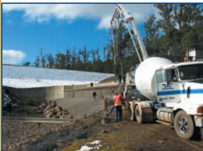
Pumping concrete with snow in the background
