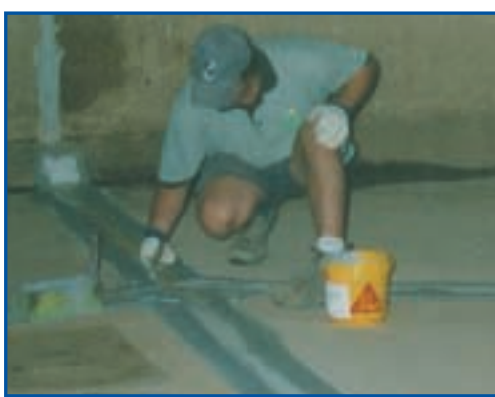
Applying Sikadur® Combiflex
