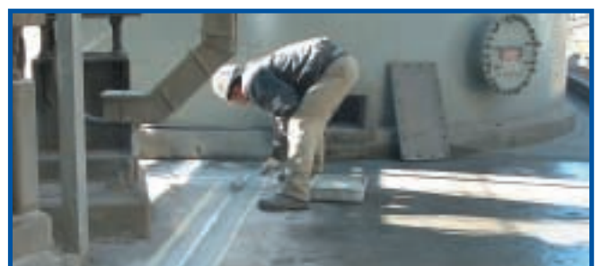
Sikagard®-62 protecting Sikadur®-Combiflex
