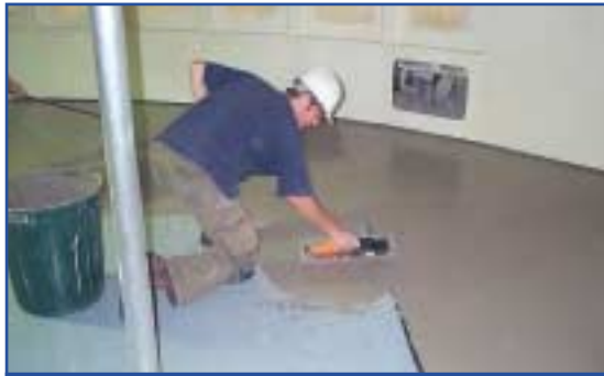
Laying the Sika Cufadan S-110
