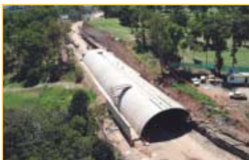
— Installation of panels
