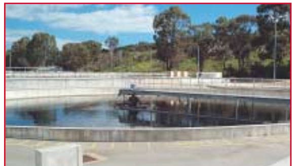
Beenyup Waste Water Treatment Plant
