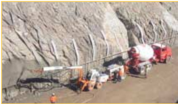
— Stratacrete and CSR spraying fibrecrete
