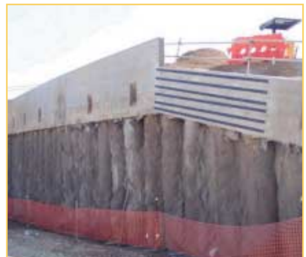
— The strengthened headstock
