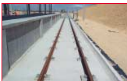
Nowergup rail line
