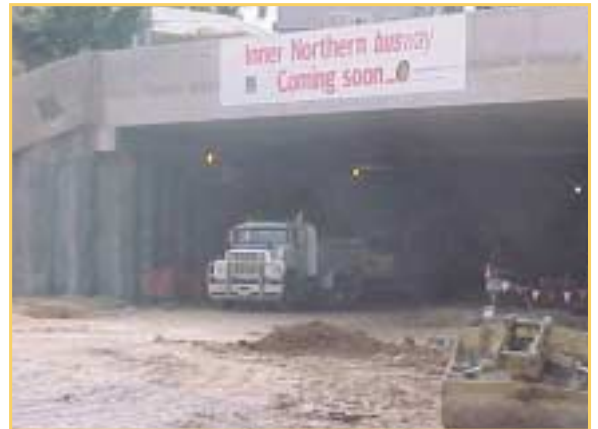
— The Inner Northern Busway construction
