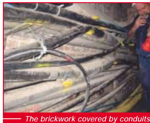
The NDC Tunnel Archway
